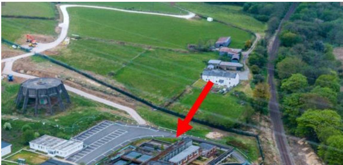
Fig. 14 - South Elevation of Brynllwarch Fawr (overlooking eastern part of Factory)
